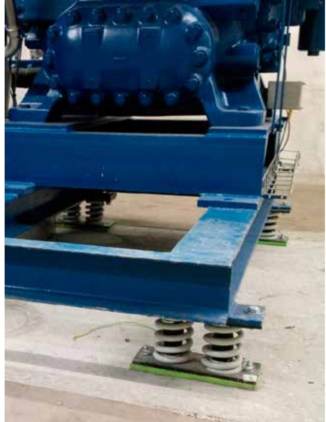
Compressor insulated with VIBRABSORBER +Sylomer®
